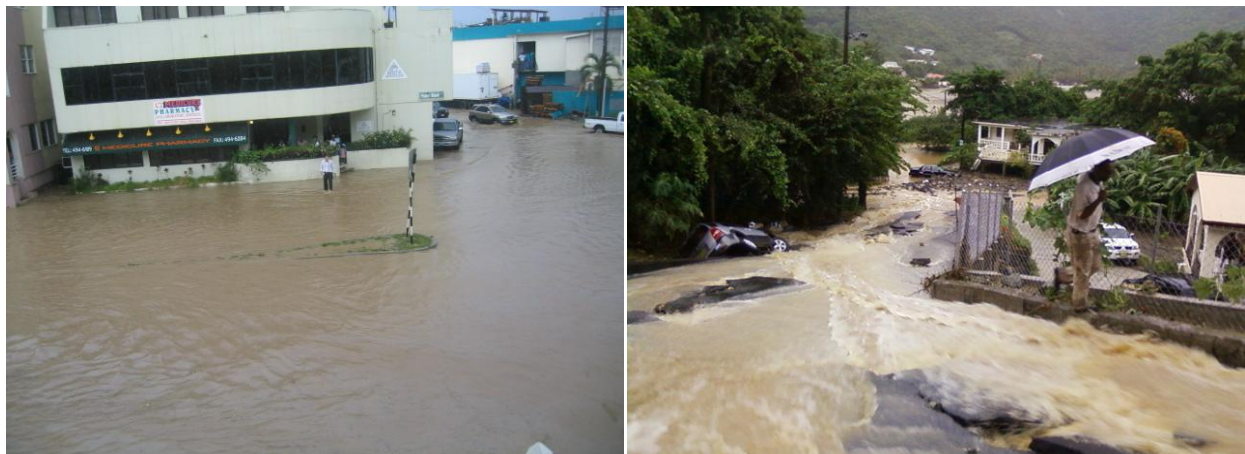
Figure 3.1-8 Some of the damage experienced in Road Town (left) and Cane Garden Bay (right) from the November 2003 and September 2010 floods.
